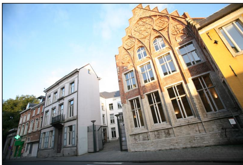
Faculty of Economics and Business - Restored historical building
